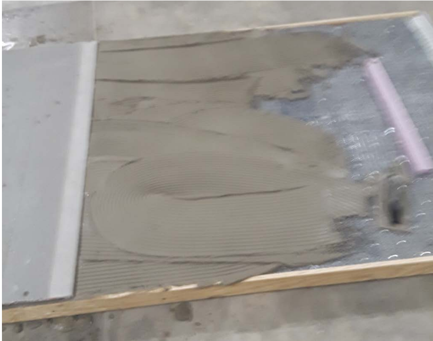
Photo No. 4 Installation of Mortar and Cement Board Layer
