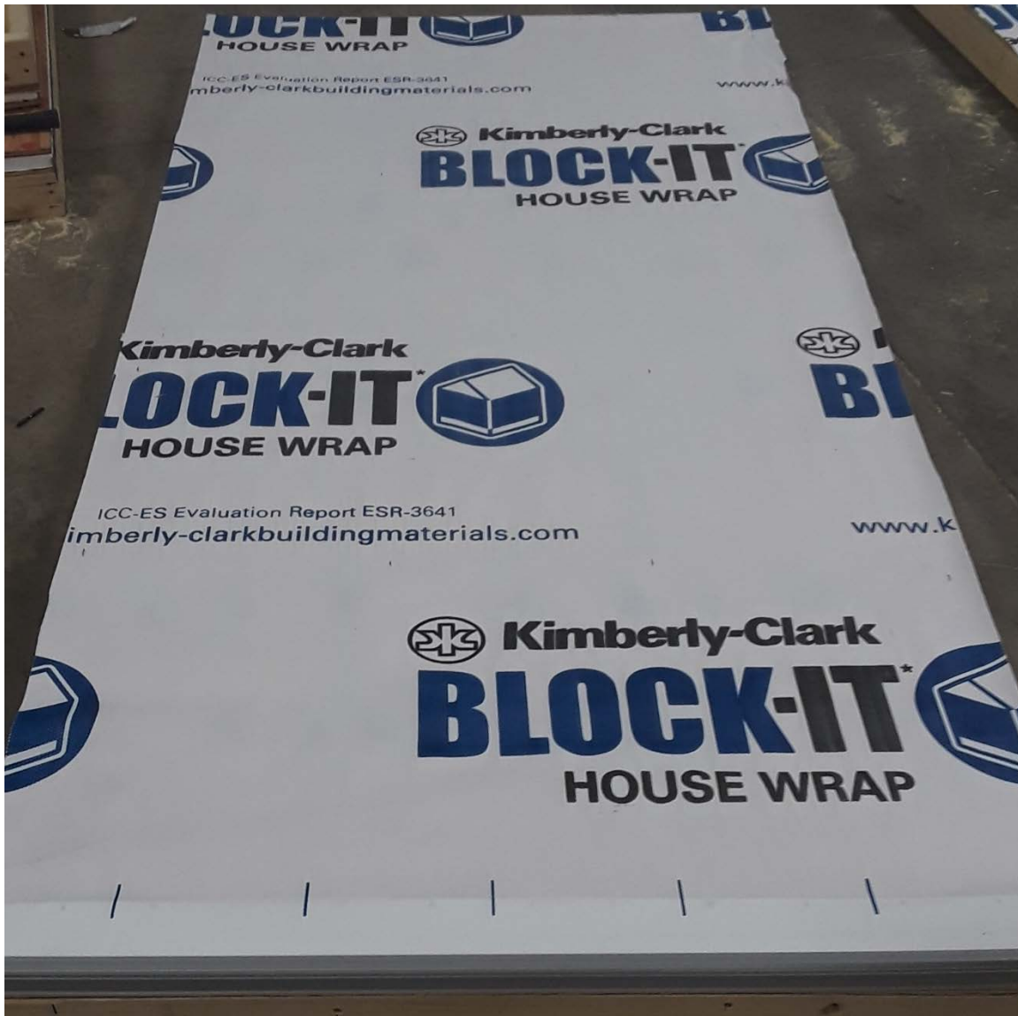
Photo No. 1 Installation of WRB Layer
