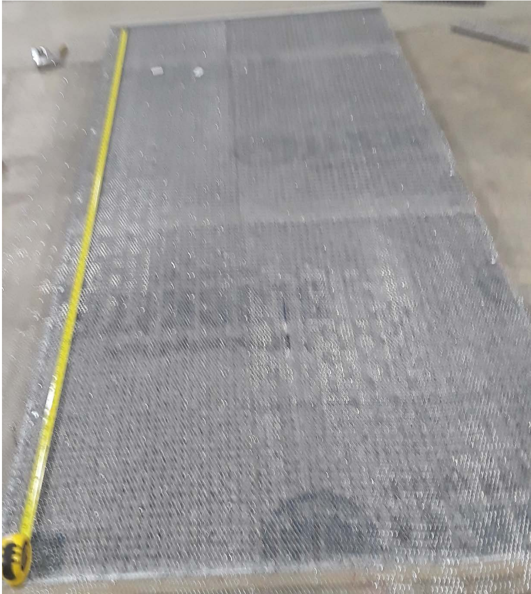
Photo No. 3 Installation of Metal Lath Layer
