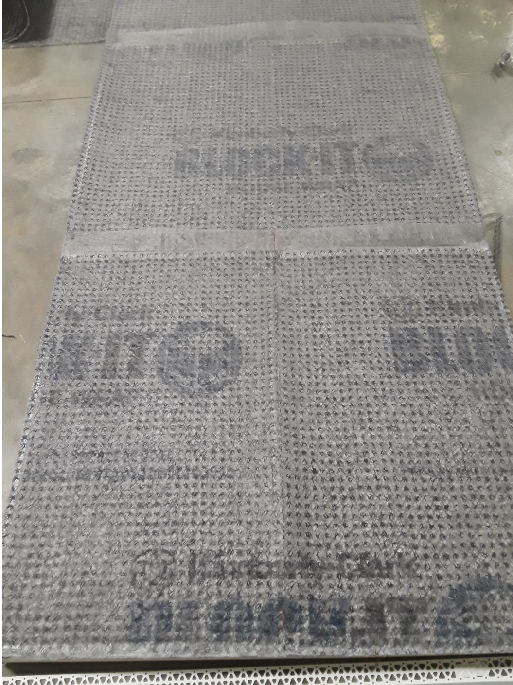
Photo No. 2 Installation of Hydrodry Rainscreen Layer
